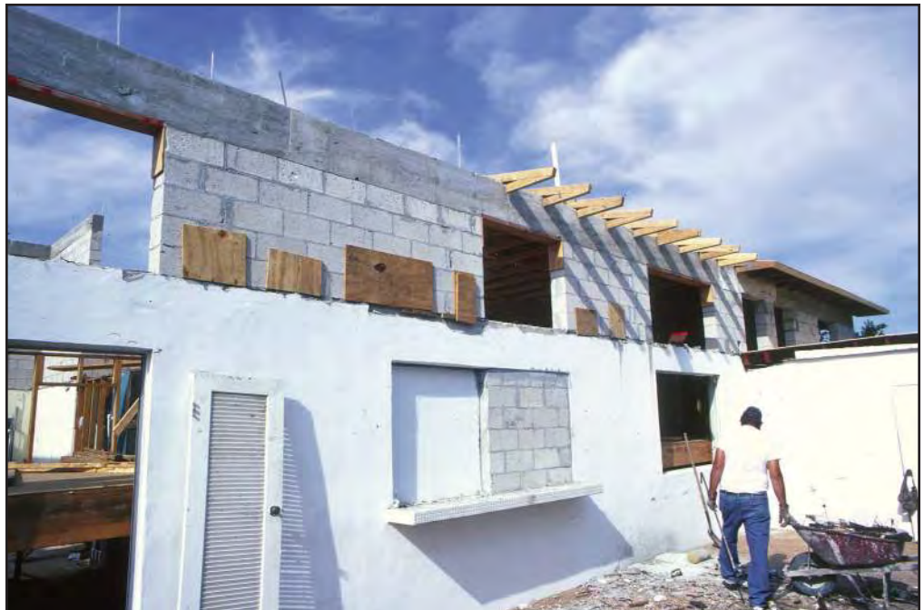
Figure 67 The extended first-story walls.
